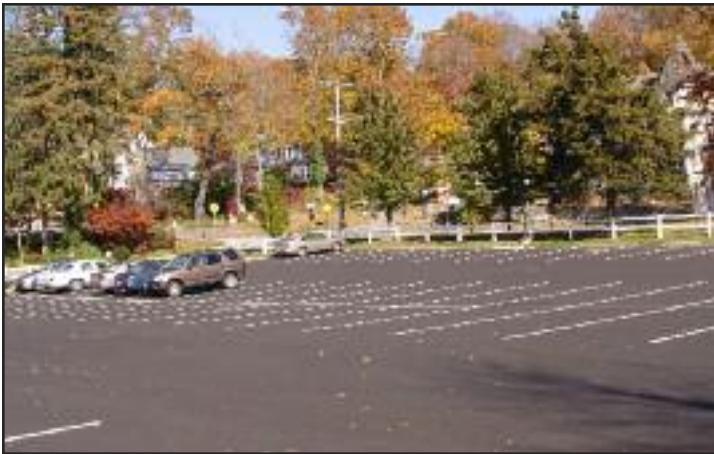
Our newly repaved and repainted parking lot thanks to the generosity of Whitney Posillico
