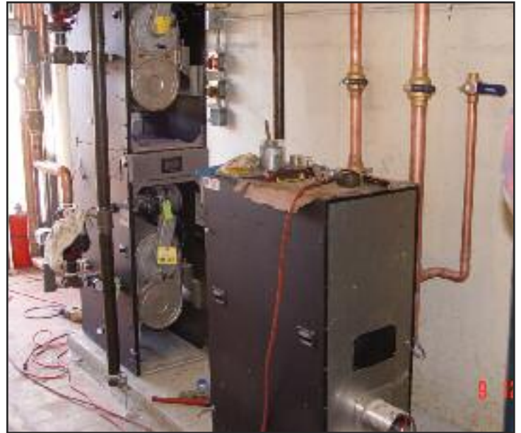
The newly installed gas heating system in the Church
