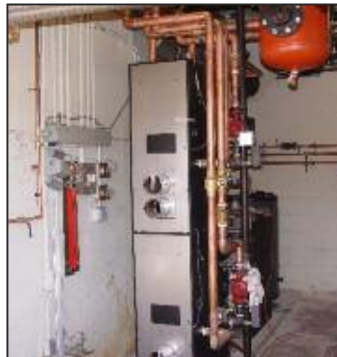
The newly installed gas heating system in the Church
